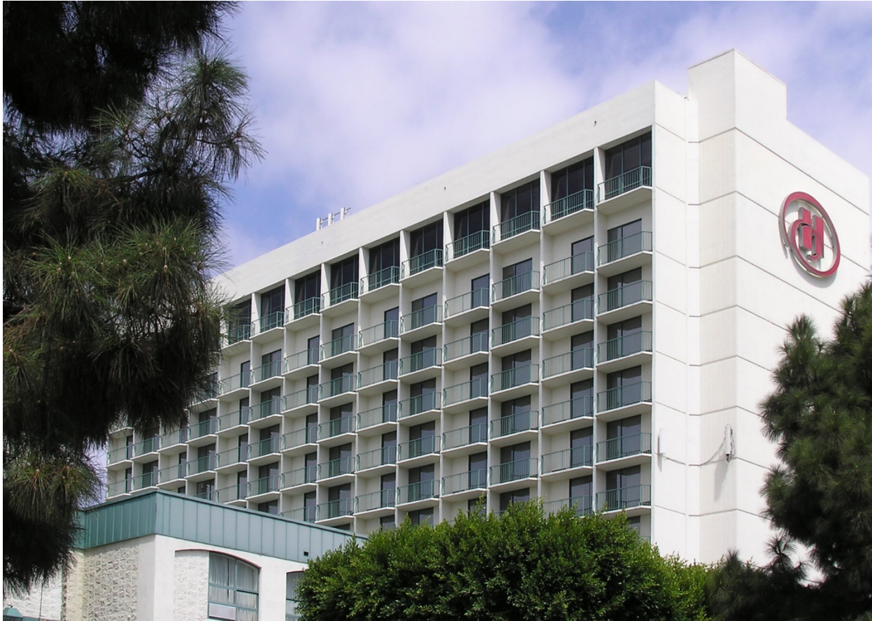
Figure 4: Hotel supporting various cellular antennas on the rooftop and sides (Torrance, CA). Photograph by Dr. Jonathan Kramer.
