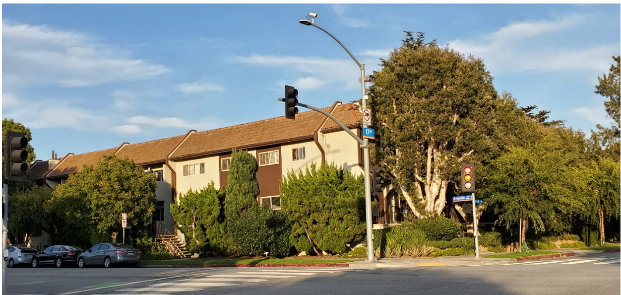
Figure 9: Single-carrier, single-band, two-sector 5G site on an existing traffic signal pole in the right of way (Santa Monica, CA). Photograph by Dr. Jonathan Kramer.
