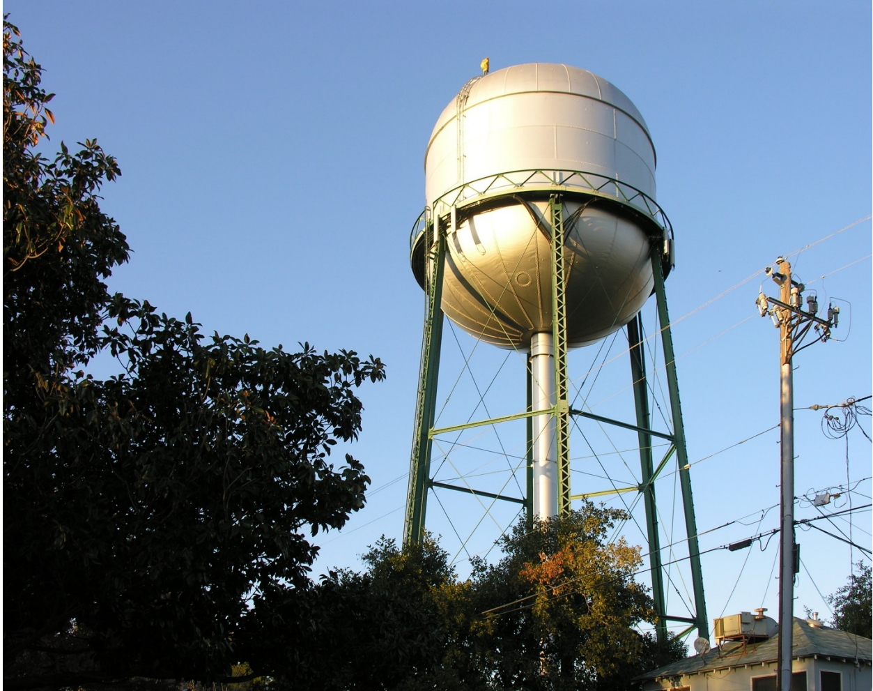
Figure 3: Lattice water tank supporting T-Mobile antennas (Chico, CA). Photograph by Dr. Jonathan Kramer.
