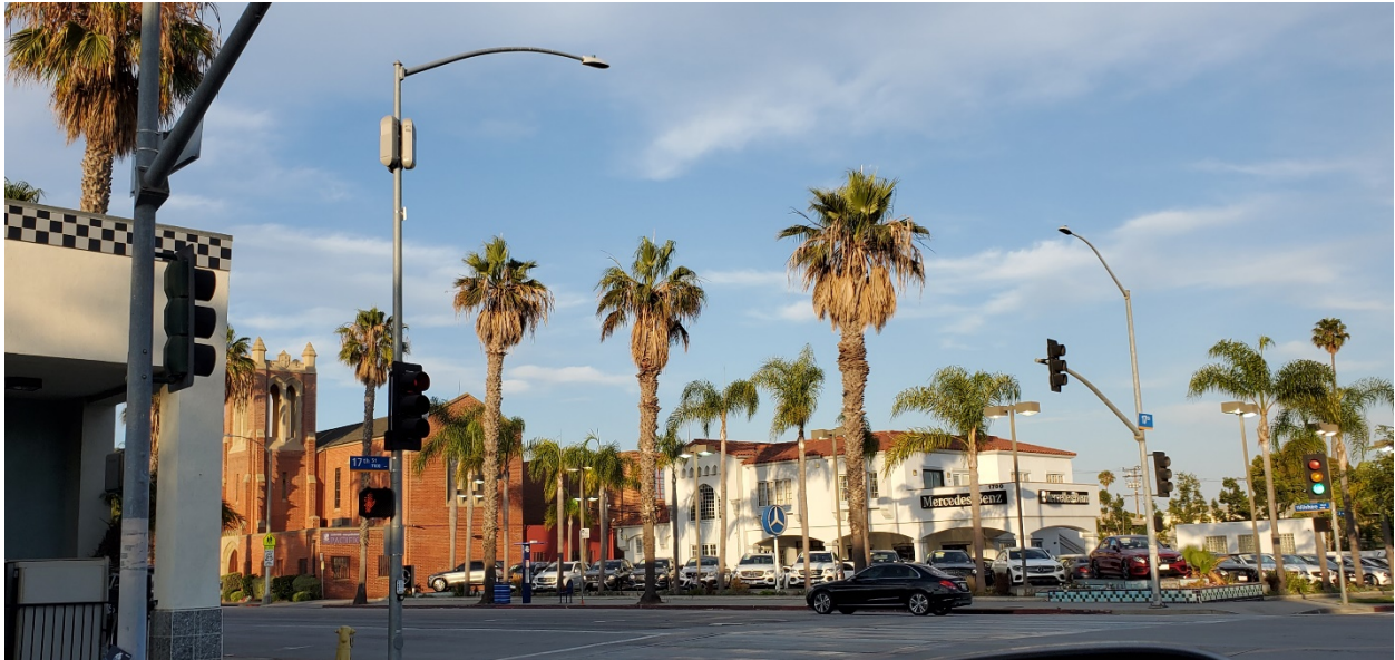
Figure 8: Single-carrier, single-band, three-sector 5G site on an existing traffic signal pole in the right of way (Santa Monica, CA). Photograph by Dr. Jonathan Kramer.
