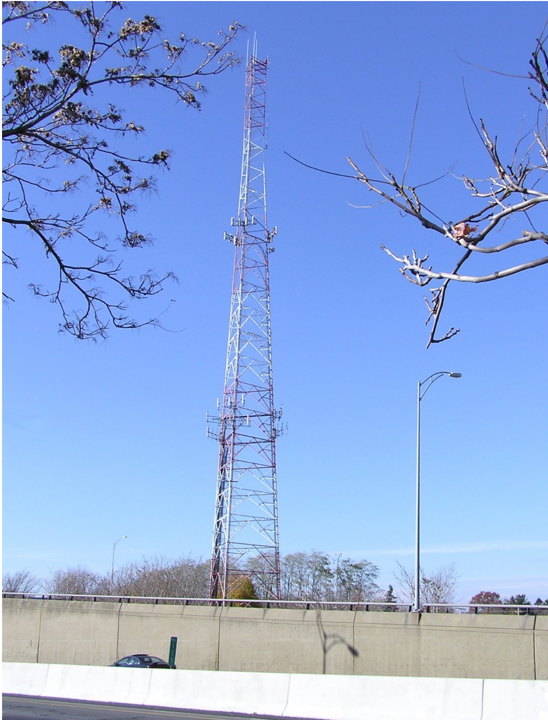
Figure 1: Self-supporting lattice tower supporting multiple cellular carriers (Newton, MA). Photograph by Dr. Jonathan Kramer.
