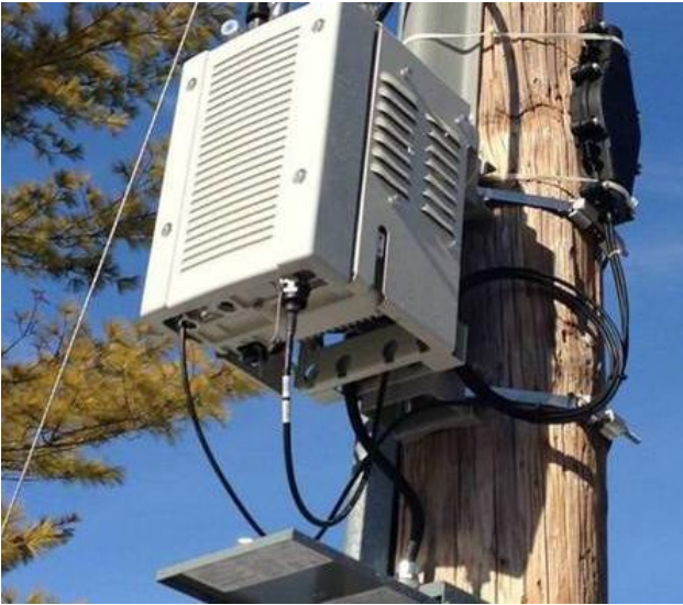
Utility Pole Mounted Antenna above
