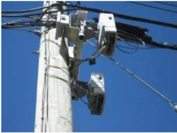
Small Cell Mounted on Telephone Pole
