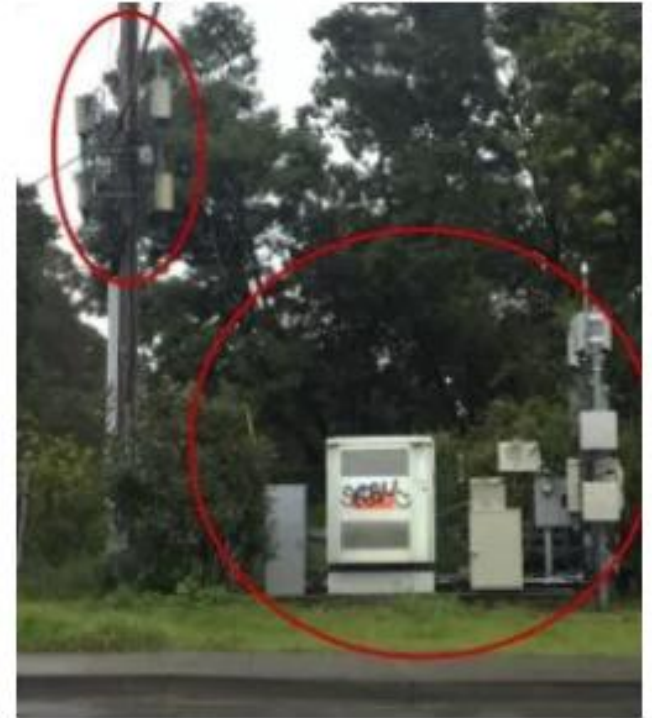
Small Cell on Pole with Power Supply Cabinet and Equipment on Ground
