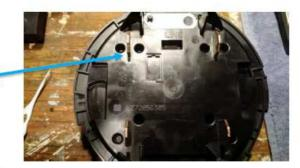
Inside of your meter box are two semicircular rings that now connect to nothing in the meter, therefore surge suppression no longer exists
