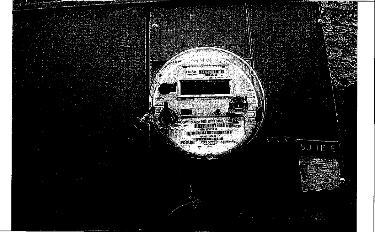
Photo No. 2: Replacement power meters (note mfg. of replacement meter is Landys + Gyr)
