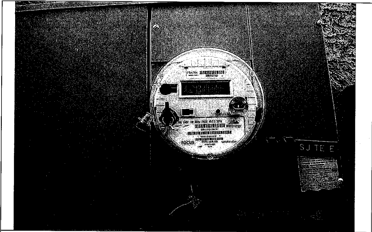
Photo No. 3: Replacement power meters (note mfg. is Landys + Gyr)
